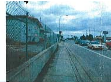
South side looking west
