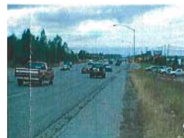
North side looking west
