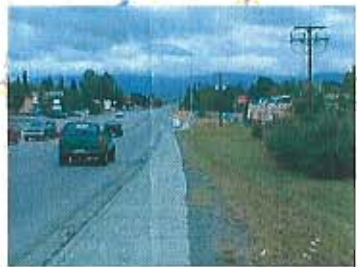
South Side looking east
