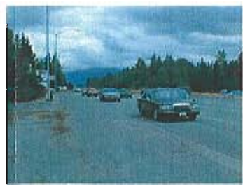
North Side looking east
