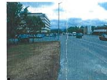
North side looking east
